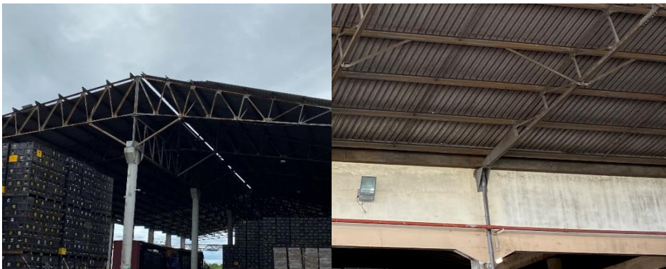
Figure 7: Un/Loading Bay (South) – Anomalies
