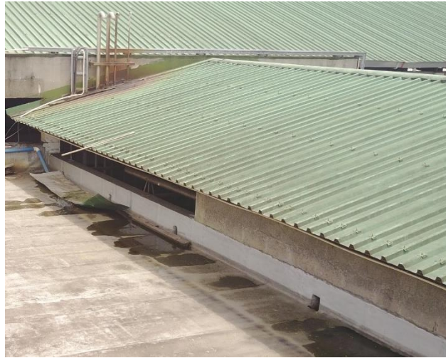
Figure 9: CO 2 Plant – Gap
