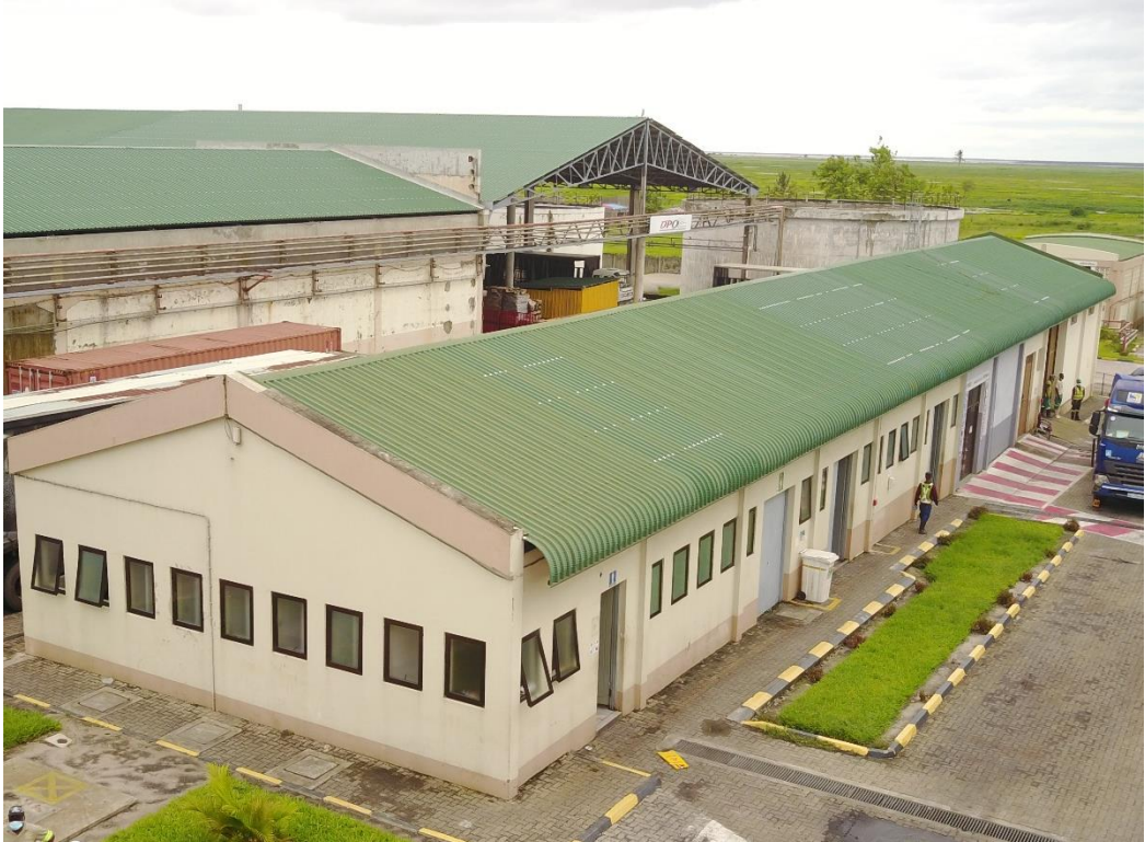
44. Change Rooms: overview
