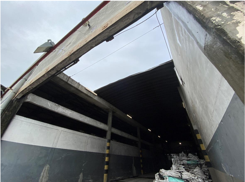
40. Roof between the empty bottles warehouse and the logistics meeting room
