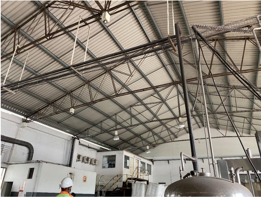
47. Old Chibuko House: roof structure in fairly good condition
