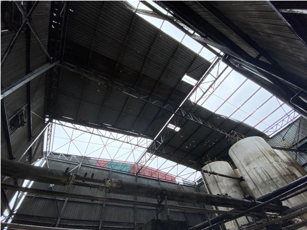
10. Old Cellars: roof view from inside the building
