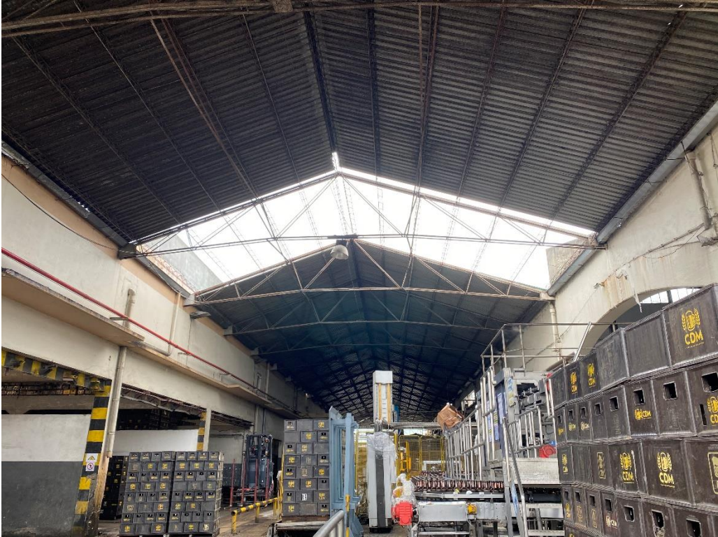
34. Pack Hall: part of the tunnel uncovered
