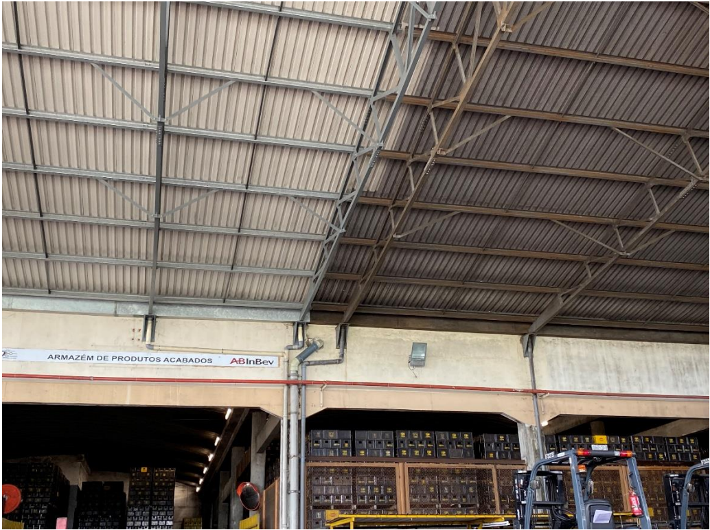
43. Un/Loading Bay: difference between the new and old roof
