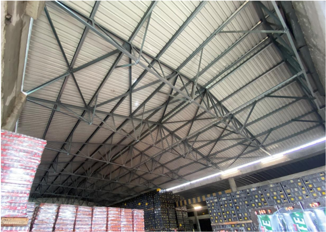
37. Fulls Warehouse: new roof structure
