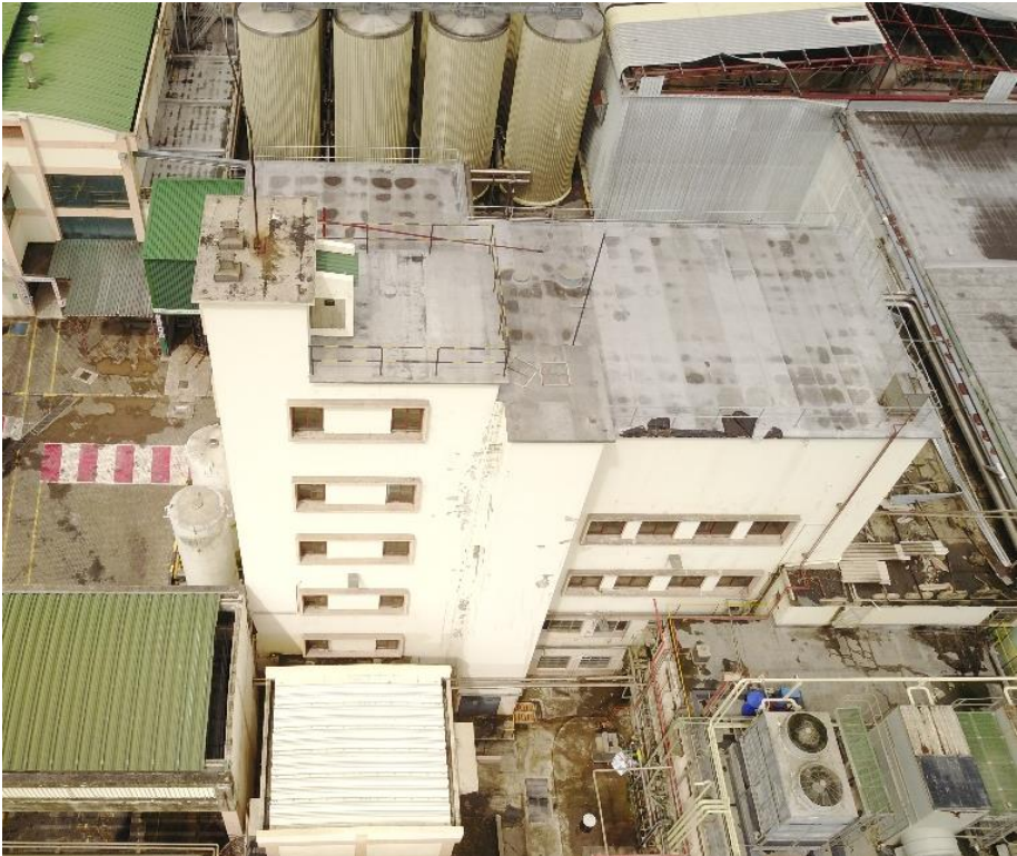
51. Silos Building: overview
