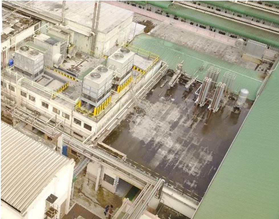
55. Engine Room: overview
